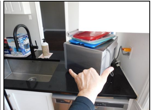
Electrical: - Outlet next to the sink not protected with GFCI. This is a safety hazard and it should be corrected to enhance safety.
