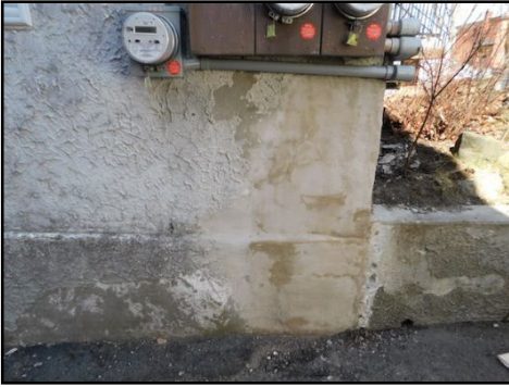
Repaired foundation area. No info provided
