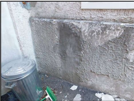
Repaired foundation area. No info provided
