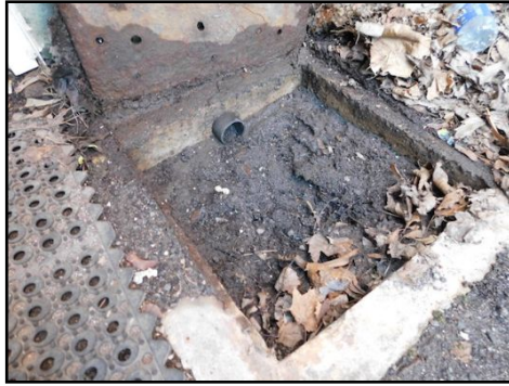
Drain Pit: Overall usable, needs cleaning.
