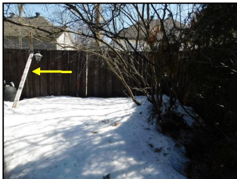
Although not part of the inspection, the rear fence is being held up by two x fours. According to the neighbor, it fell over.
