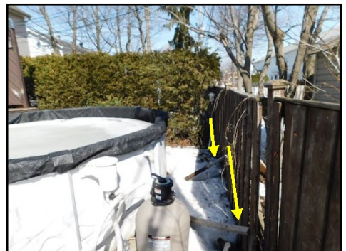
Although not part of the inspection, the rear fence is being held up by two x fours. According to the neighbor, it fell over.
