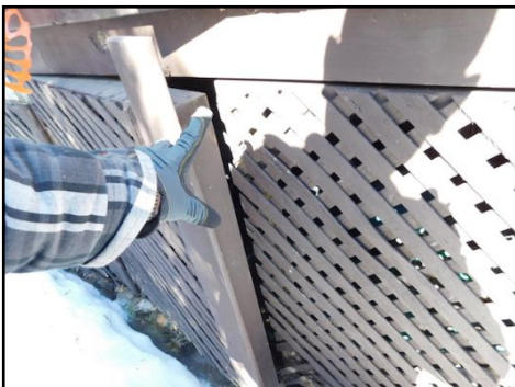
Not verifiable underneath due to snow/ice
